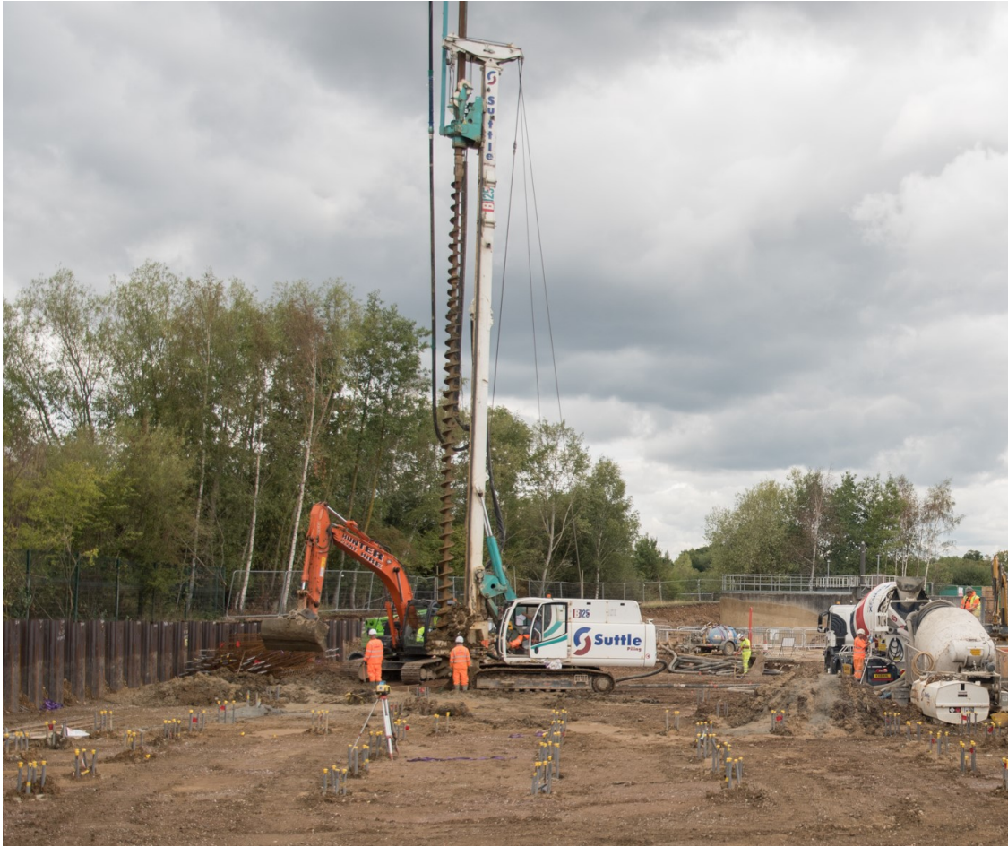
Piling with our Casagrande B125 piling rig
